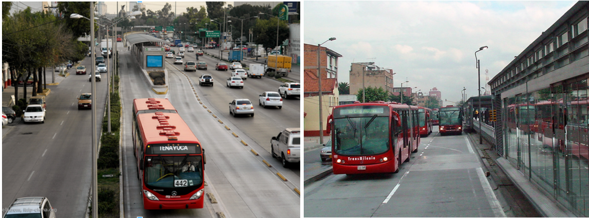
Figure 3: A single-lane BRT system like that in Mexico City (left) can handle volumes from 5,000 to 15,000 pphpd. With passing lanes at stations, a BRT system can carry up to 45,000 pphpd, the capacity of Bogotá's TransMilenio (right).
