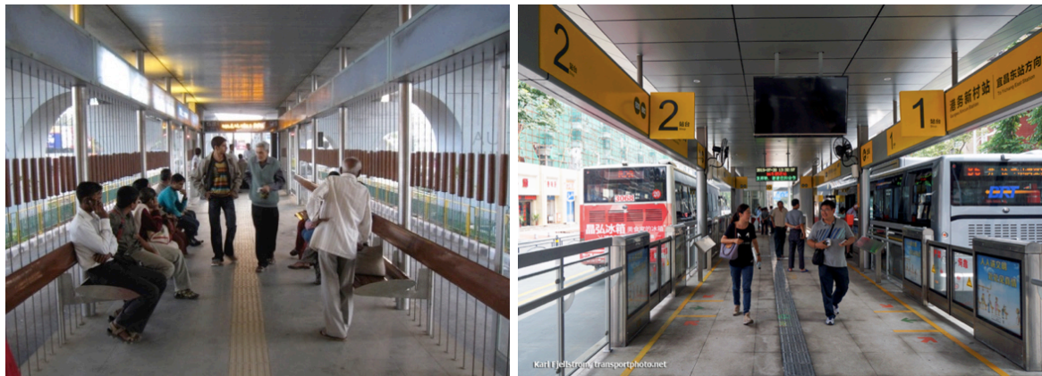
Figure 31: Passive solar design provides shading and encourages natural ventilation: Janmarg, Ahmedabad, India (left) and Yichang BRT, China (right).
