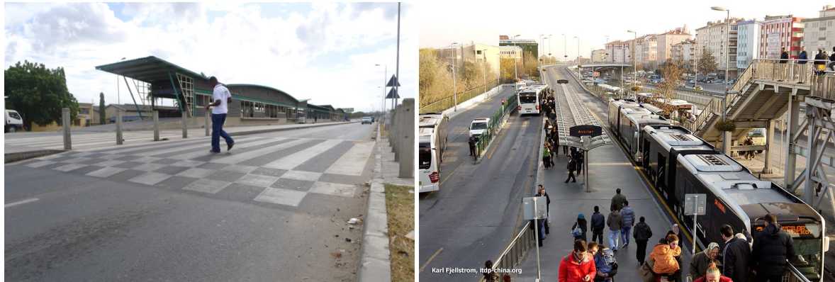
Figure 29: Safe at-grade pedestrian crossings, such as the speed table crossings in Dar es Salaam (left), are preferred as they provide easy, convenient access to BRT stations. On highway corridors such as in Istanbul (right), foot overbridges can be considered provided they have adequately sloped ramps or working escalators or elevators.
