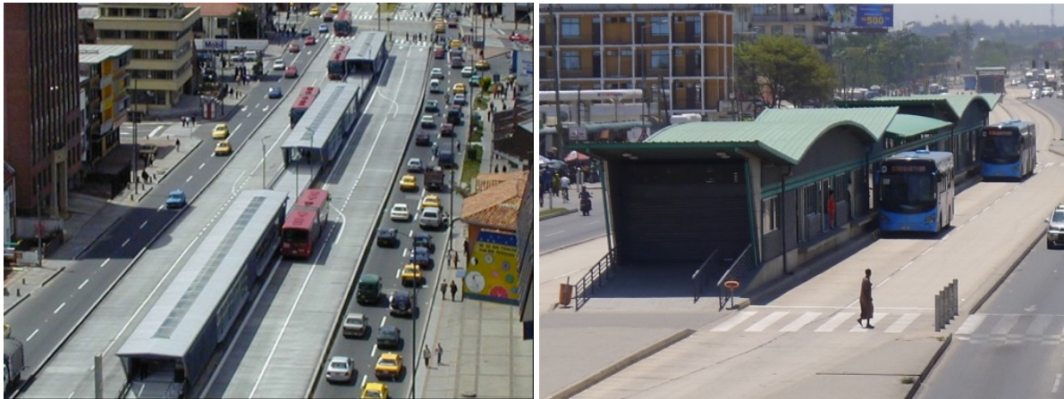
Figure 7: Stations with multiple sub-stops in Bogotá (left) and Dar es Salaam (right) increase system capacity and speed. A gap of 1.8 times the bus length is required between sub-stops to allow buses to pass other vehicles that are stopped for boarding and alighting.
